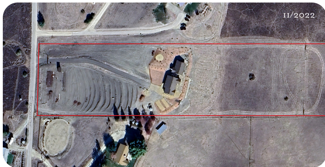
Preparatory stages of farm development: Grading, Irrigation install
